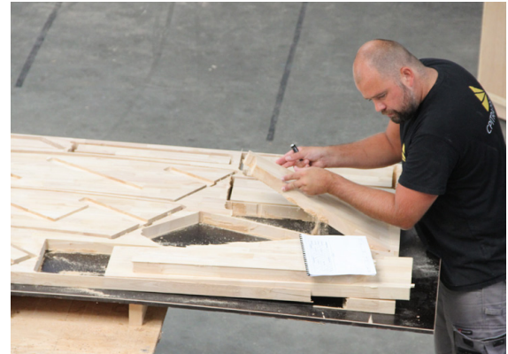
While the machine is running, the operator has time to remove parts from the previously finished plate and label them.
